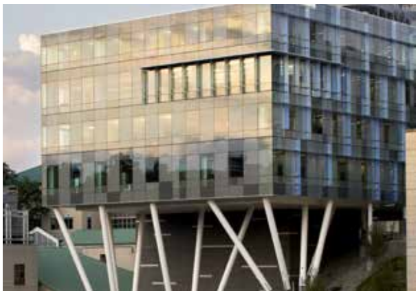
D-M Products fabricated, supplied, and installed the dichroic glass curtain wall at Carnegie Mellon's Scott Hall. Photo by Jeremy Bittermann.
